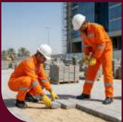
ROAD WORKS (ASPHALT, INTERLOCK, CURBSTONES)
