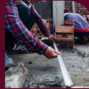
SITE GRADING & LEVELING
