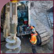
EARTH WORKS & EXCAVATIONS
